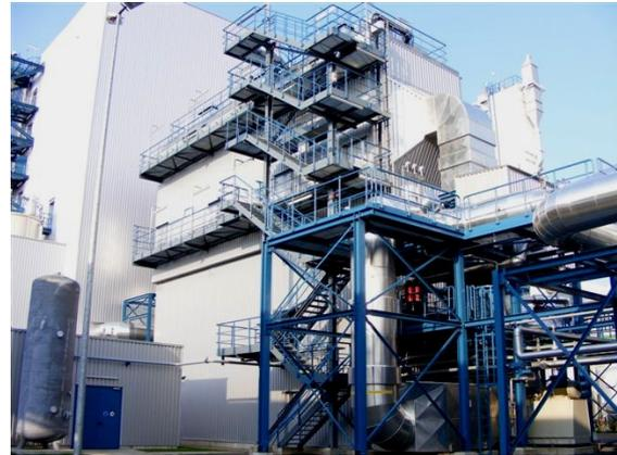
Fig. 2: Photograph of the three-field ESP at Schwarze Pumpe.
