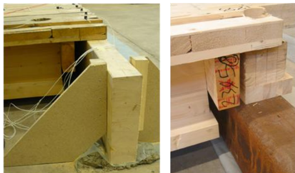
Figure 3. Simply supported support conditions in laboratory tests, floor placed on glulam beam in left picture and on steel beam in the right picture.
