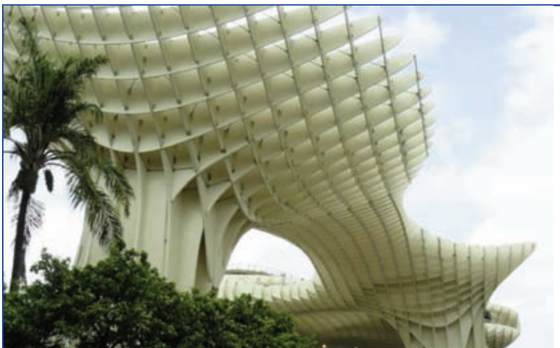
Figure 1: Metropol Parasol in Sevilla, Spain, one of the worlds largest timber engineering constructions with 3400 individual wooden elements
