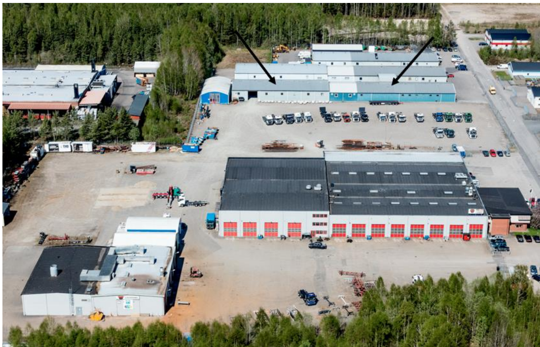
Figure 14: An overview of the company GEHAB and its surrounding area. The rooftop that is investigated is marked with arrows.
