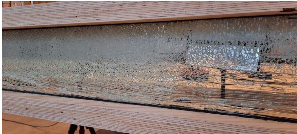
Figure 21: Crack patterns of beams with double-layer heat-strengthened glass.
